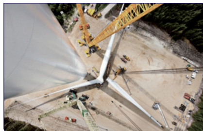
Wind turbine installation
